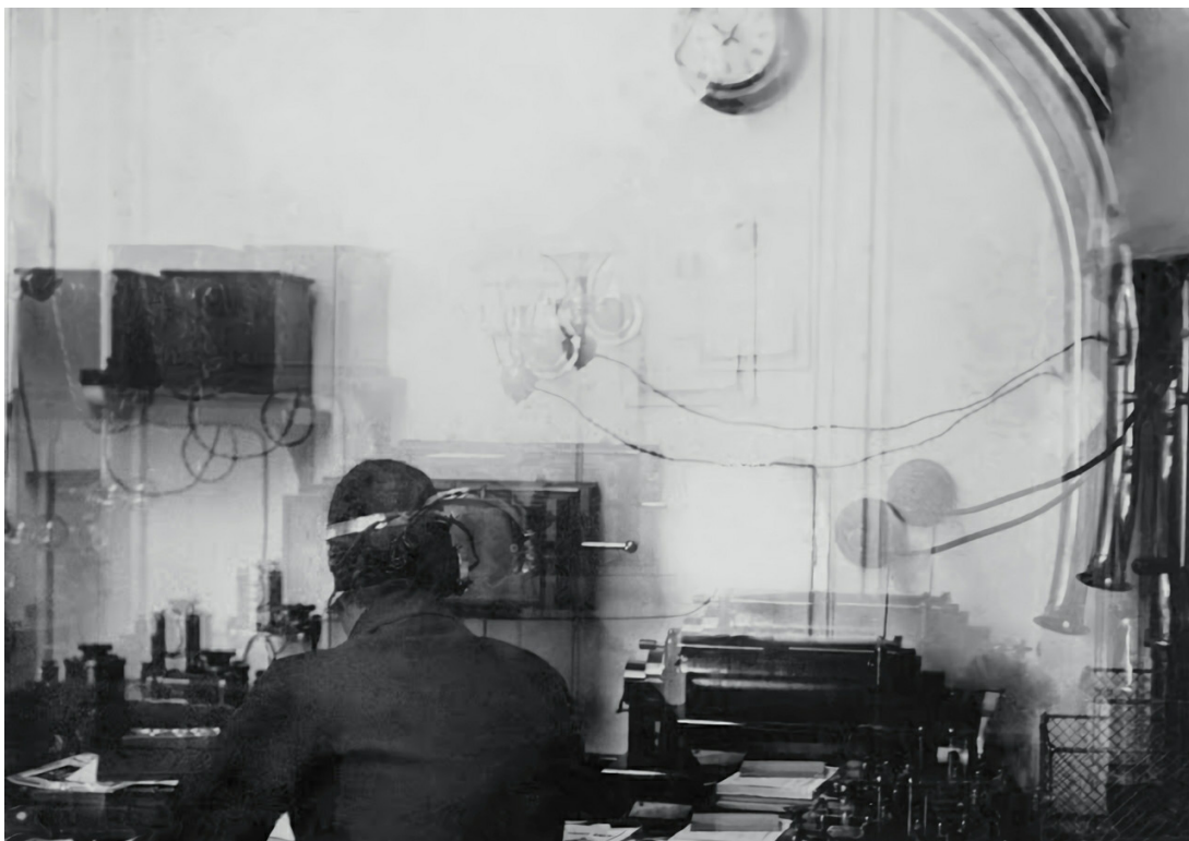
Wireless Radio room
